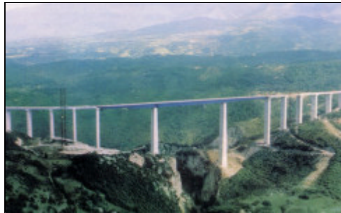
Pont Italia Bridge, Italy
