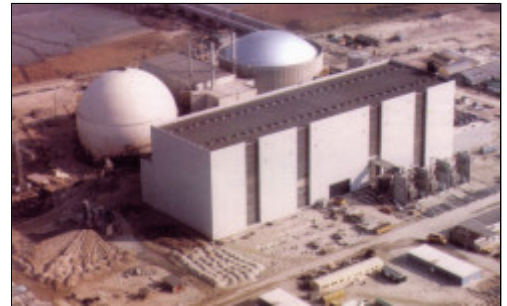
Nuclear Reactor Doel, Belgium
