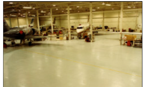
Gulfstream Hangar, Savannah
